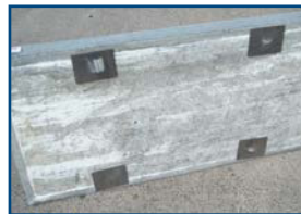
3. Insert all 4 base plates through the light weight slab and reposition to the required location of the ASHP unit.
