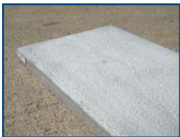
1. Position the light weight slab in the required location of the ASHP unit.
