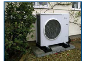
5. Secure the ASHP units onto the kit - the installation is complete.
